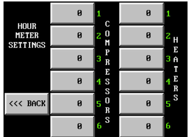
18. Compressor & Heater Hour Meter Adjustments
